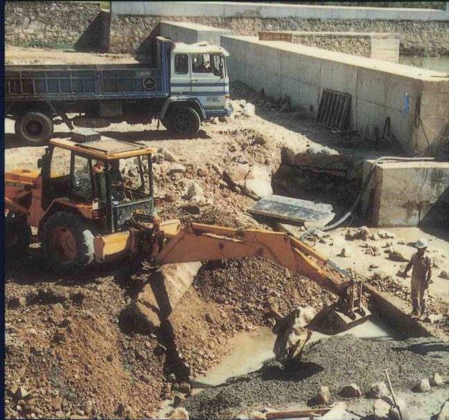
Construction of a canal measurement station
