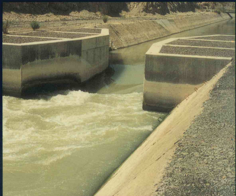
Canal structure for flow measurement.
