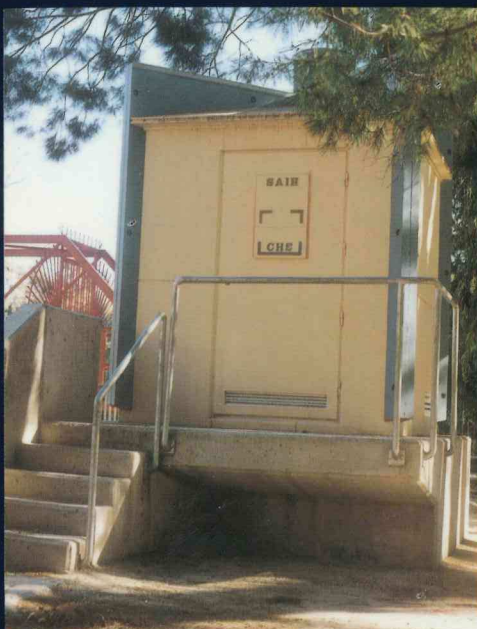
Close-up view of an elevated instrument shed.
