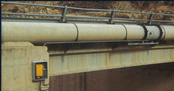
Measurement in pipe
