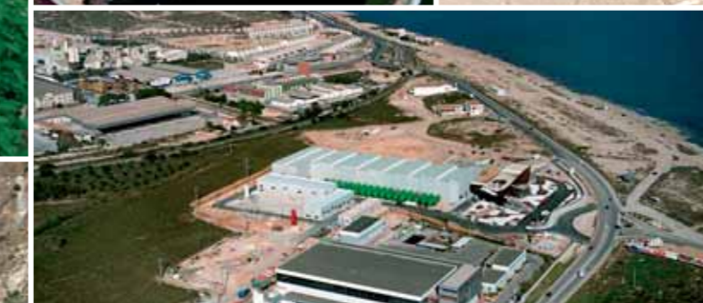
Desalination Plant Alicante 1 (Alicante), for urban supply
